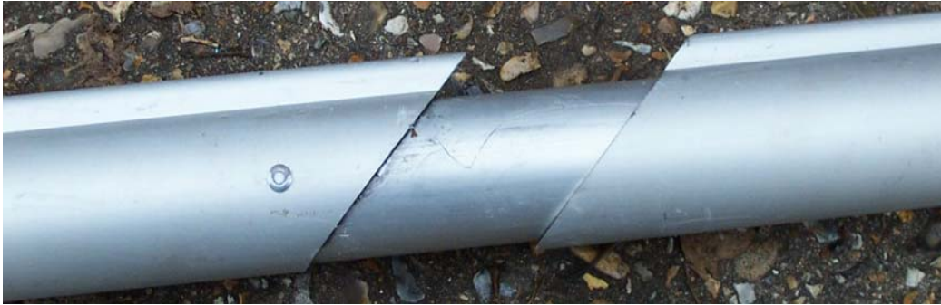
Picture 4.5 Joining the Mast
